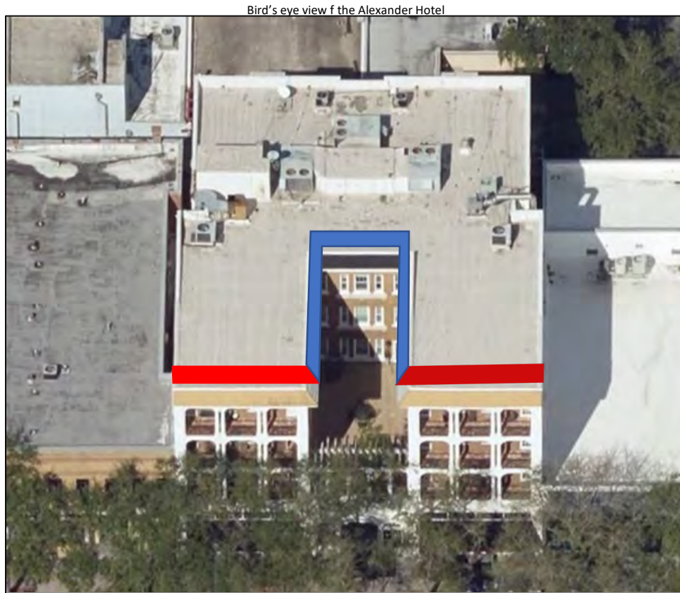
Figure 3: Bing bird's eye view of the Alexander Hotel. The mansard roof in red is the portion of roof with asbestos tile. The mansard roof in blue is the portion of roof with French-style tile. The entirety of the mansard roof would have originally been clad with a French-style tile.
