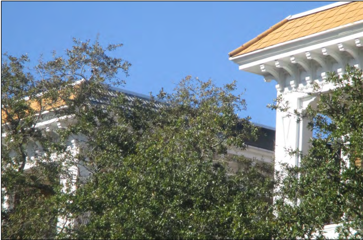
Figure 4: 2018 photograph by staff of the Alexander Hotel, showing flat roof tile on front elevations of mansard roof and grey textured tile on inner mansard roof portions.
